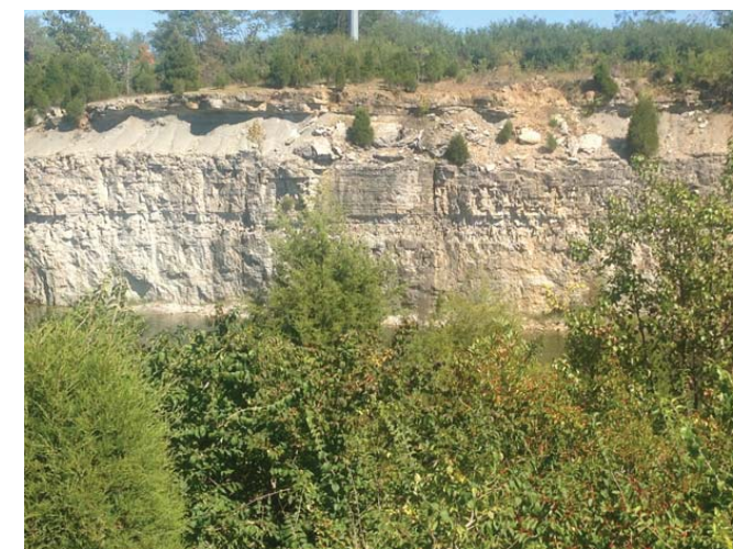
Quarry high wall – flooded pit. Highly erodible and problematic Waldron shale cap.
